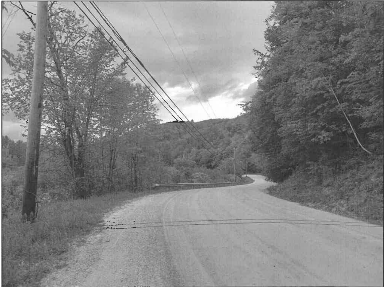
Northbound view of River Road, about 400 ft. north of Thundering Brook Road shown here with an Automatic Traffic Recorder with its tubes installed across the road surface, May 2022.
